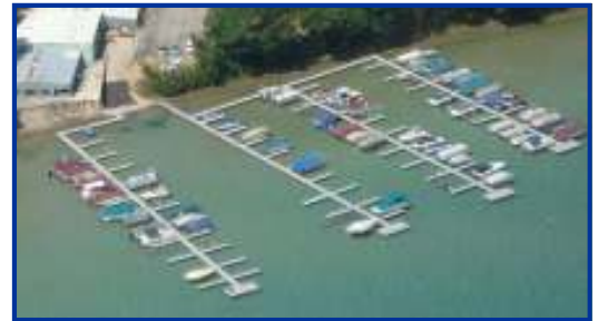
Aerial view of new marina Custom supplied per association specifications
