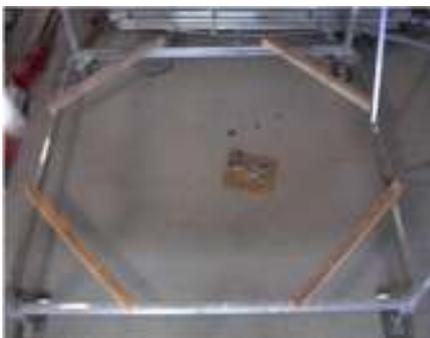
(7) Lay (4) 4 x 4's or any 4 equal size boards diagonally across each corner. This will make it easier to put the lift carriage together in the next step.
