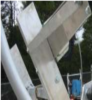
Pontoon arm installation.
