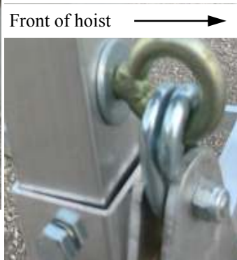
Side panel upright pulley installation 1/2 x 6 Pulley Assemblies
