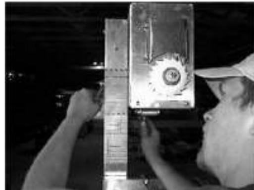
Tighten bolts like above pictures 9/16" socket on inside and 9/16" open end wrench on outside.
