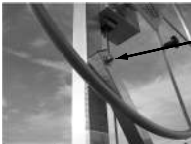
Close up of winch column brace connection.
