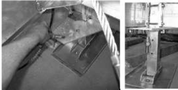
View of non winch column front of hoist
