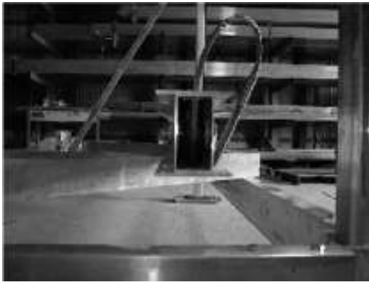
End view of twin beam on non winch side of hoist front. Showing longer cable fitting. That goes up.
