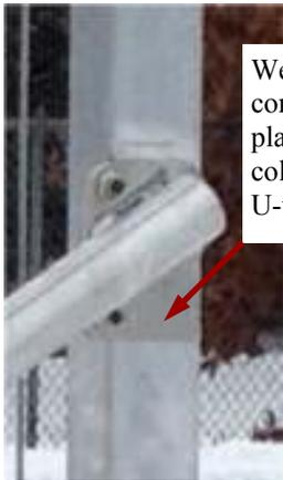
Welded connection plate on columns and U-tube
