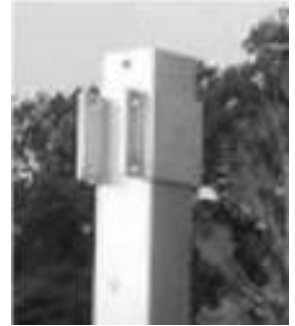
View of Non-Winch Column kitty corner from Winch Column
