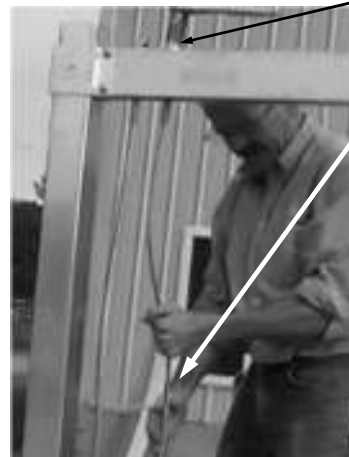
Non Winch Column front corner
